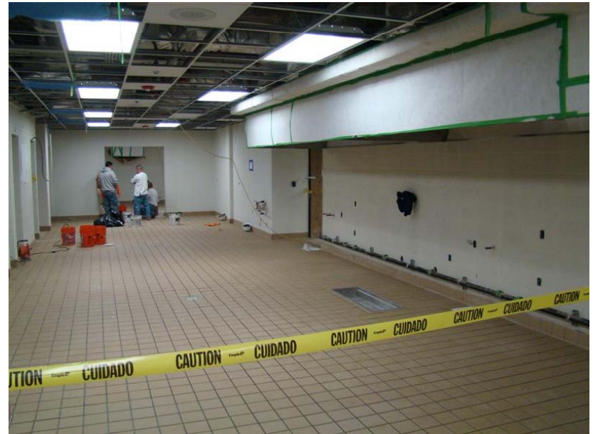
Quarry Tile Installation at Kitchen
