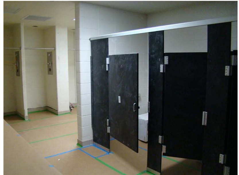
Typical Locker Room Toilet/Shower Area
