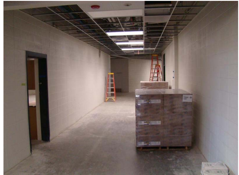
Corridor at Science Wing
