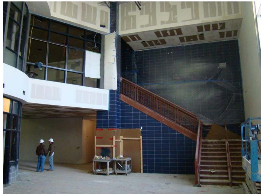
Staircase to 2 nd Level Learning Communities
