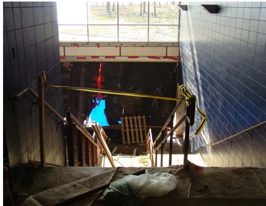
Grand Staircase View from Second Floor
