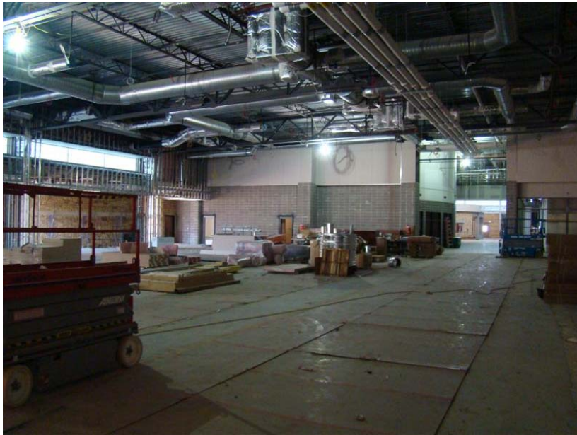
View of Cafeteria from Kitchen
