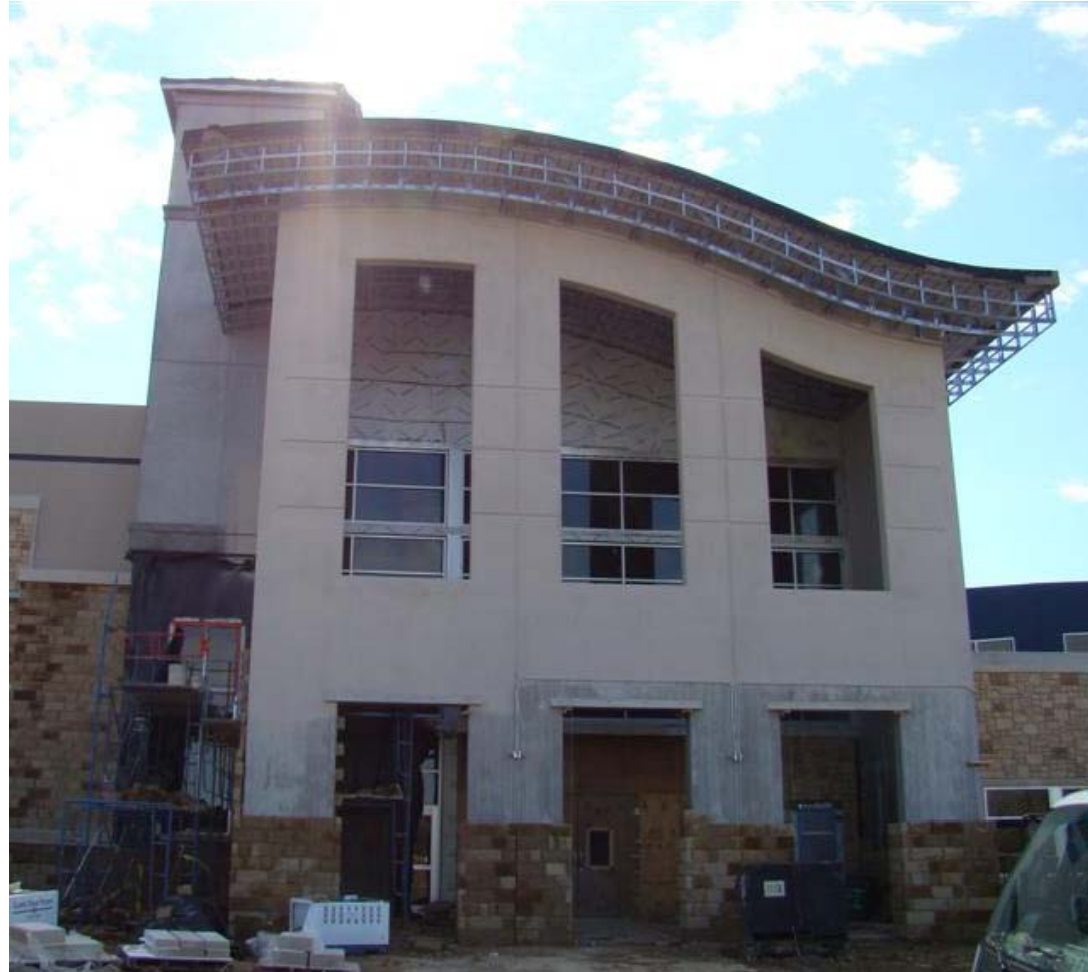
Exterior View of Main Entrance
