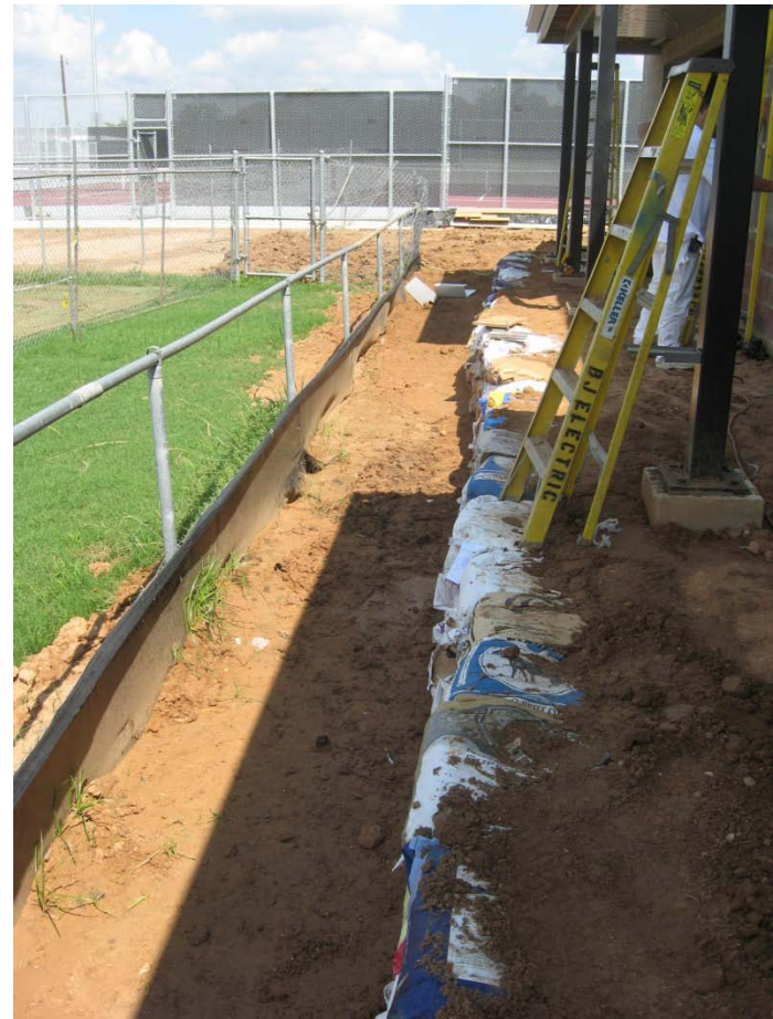
Concessions Building Work in Progress - Flatwork
