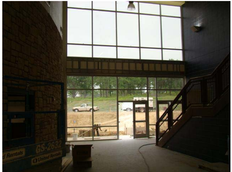
View at Entrance at Bus Loop
