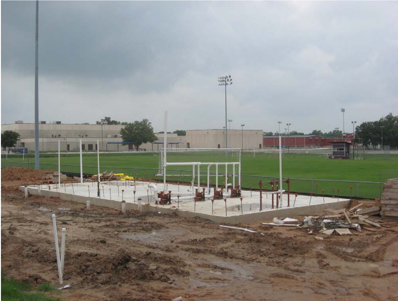
Concessions Building Rough-in Plumbing Installed
