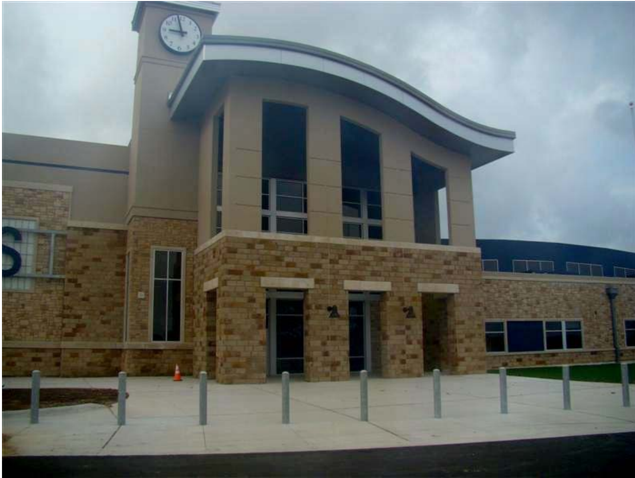
Exterior View of Main Entrance
