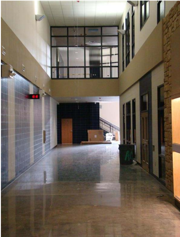
Corridor View adjacent to Library
