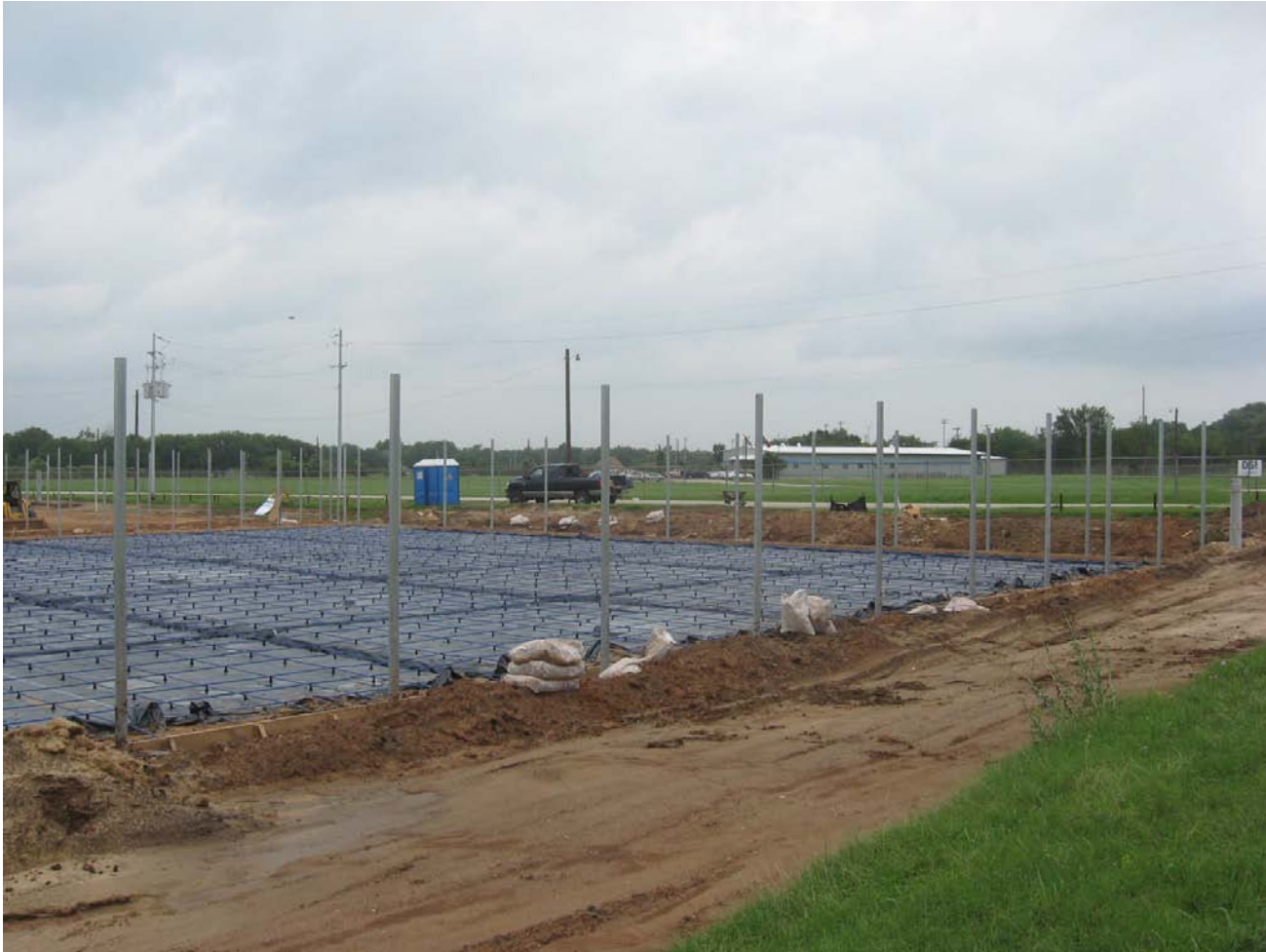
Tennis Court Post Tension Cables Section One North View
