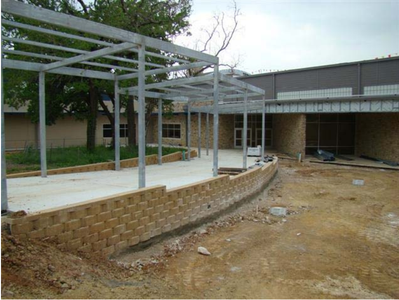
Exterior Courtyard at Bus Loop
