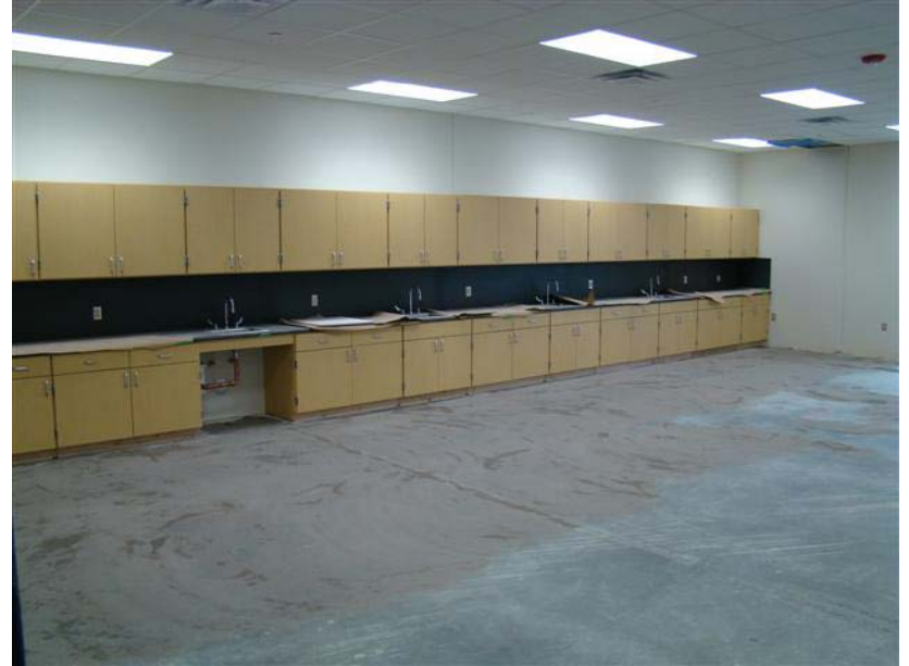
Millwork at Art Room
