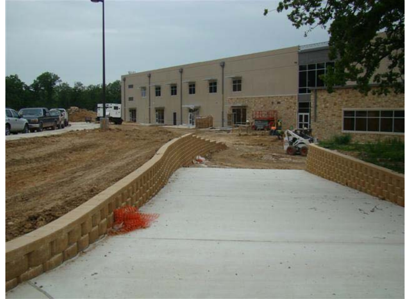
Exterior Courtyard at Bus Loop
