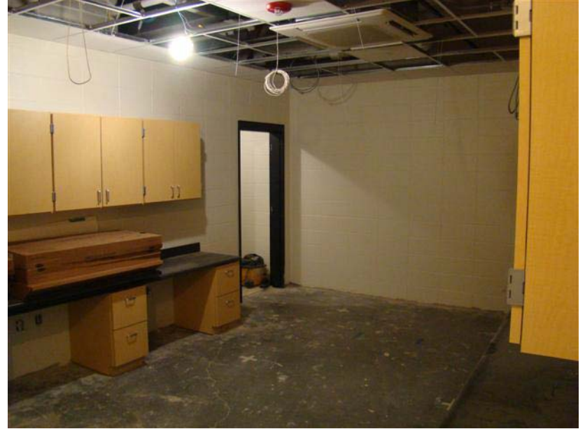
Millwork at Coaches Office
