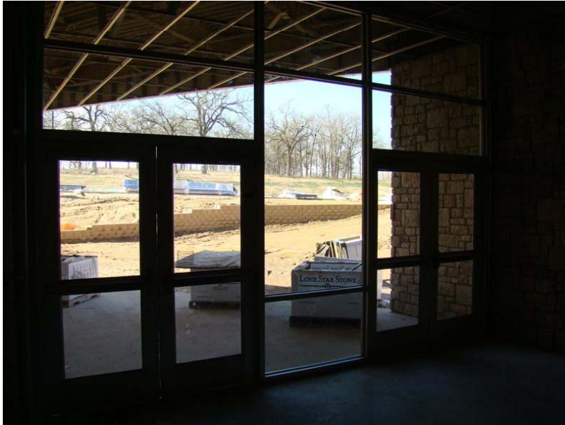
View at Cafeteria – Bus Loop Courtyard
