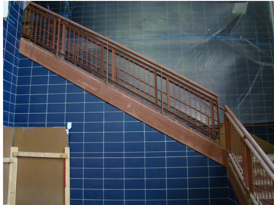
Staircase to 2 nd Level Learning Communities
