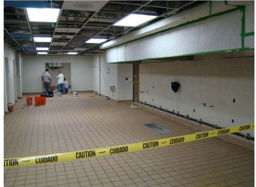
Quarry Tile Installation at Kitchen
