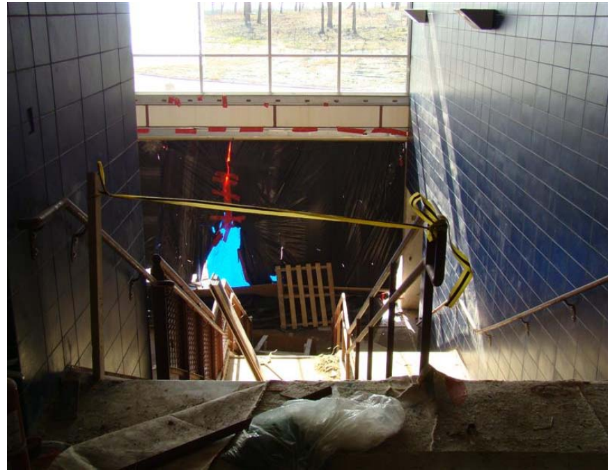
Grand Staircase View from Second Floor
