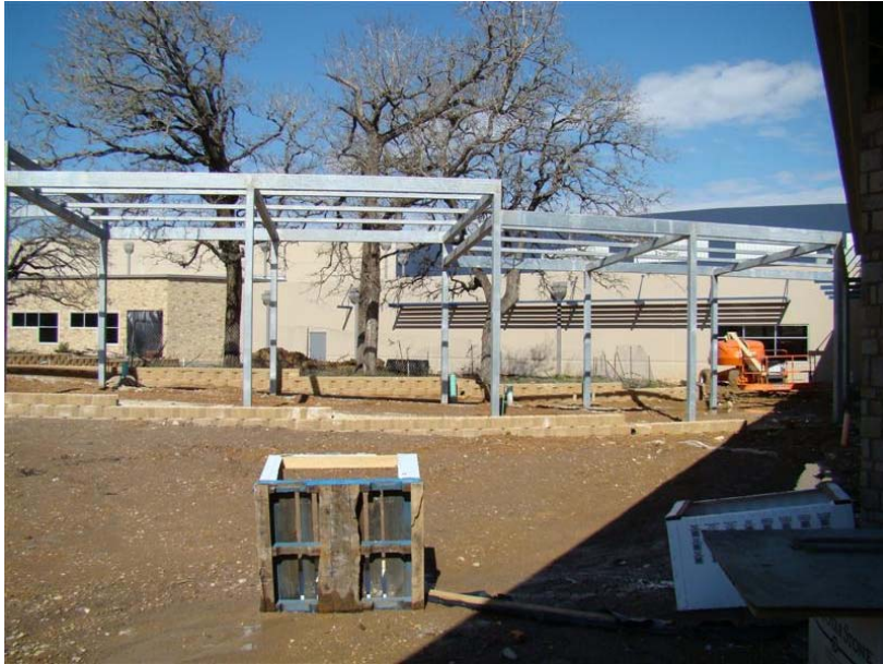
Exterior Courtyard at Bus Loop
