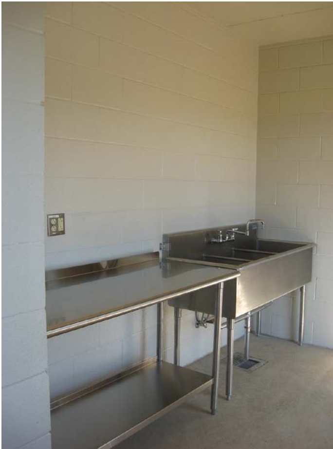
Interior Concessions 3 Compartment Sink and Stainless Steel Work Table
