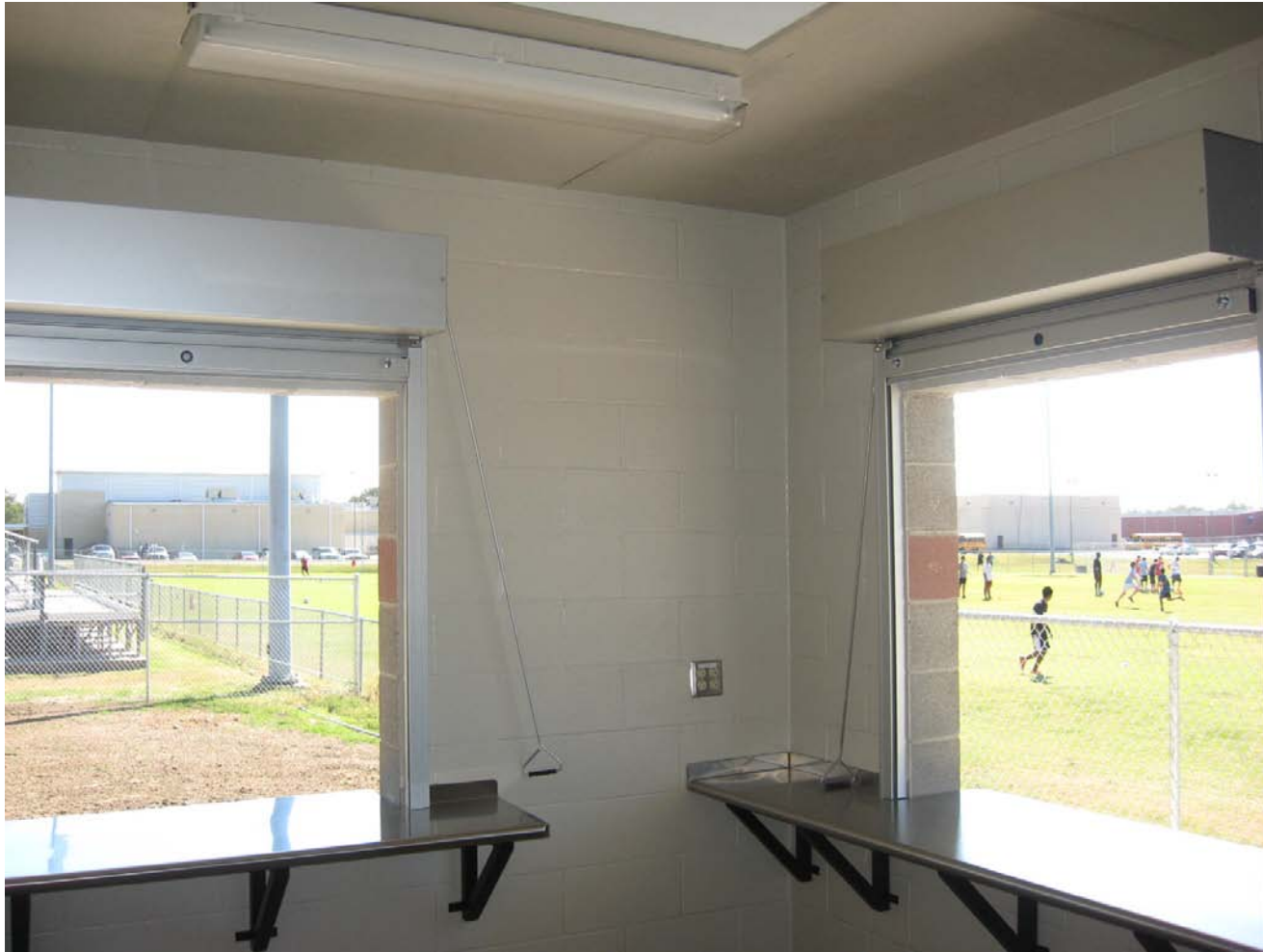
View of Soccer Field from Inside Concessions at Roll Up Service Doors
