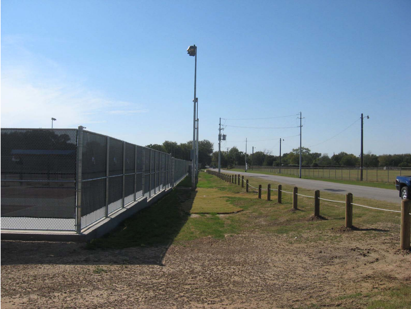
Final Grading and Hydromulch West View - Hawthorn
