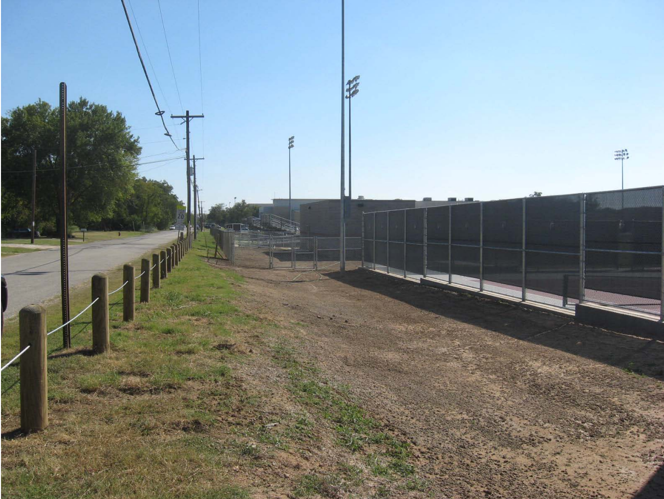
Final Grading and Hydromulch South View - Chambers
