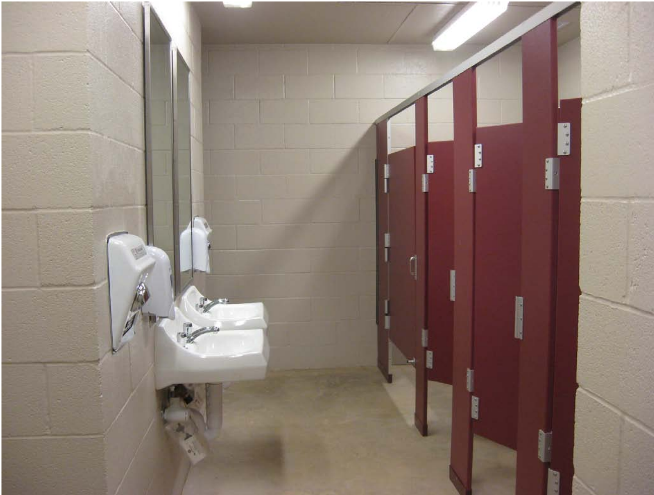
Interior Concessions at Women's Restroom
