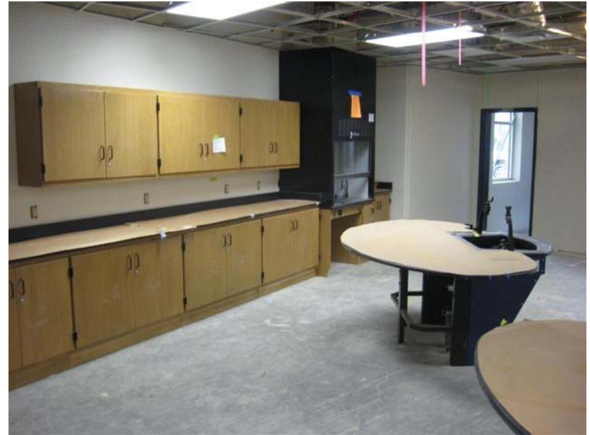
Science Casework Installation
