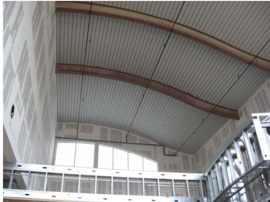
Roof Structure at Lobby Area
