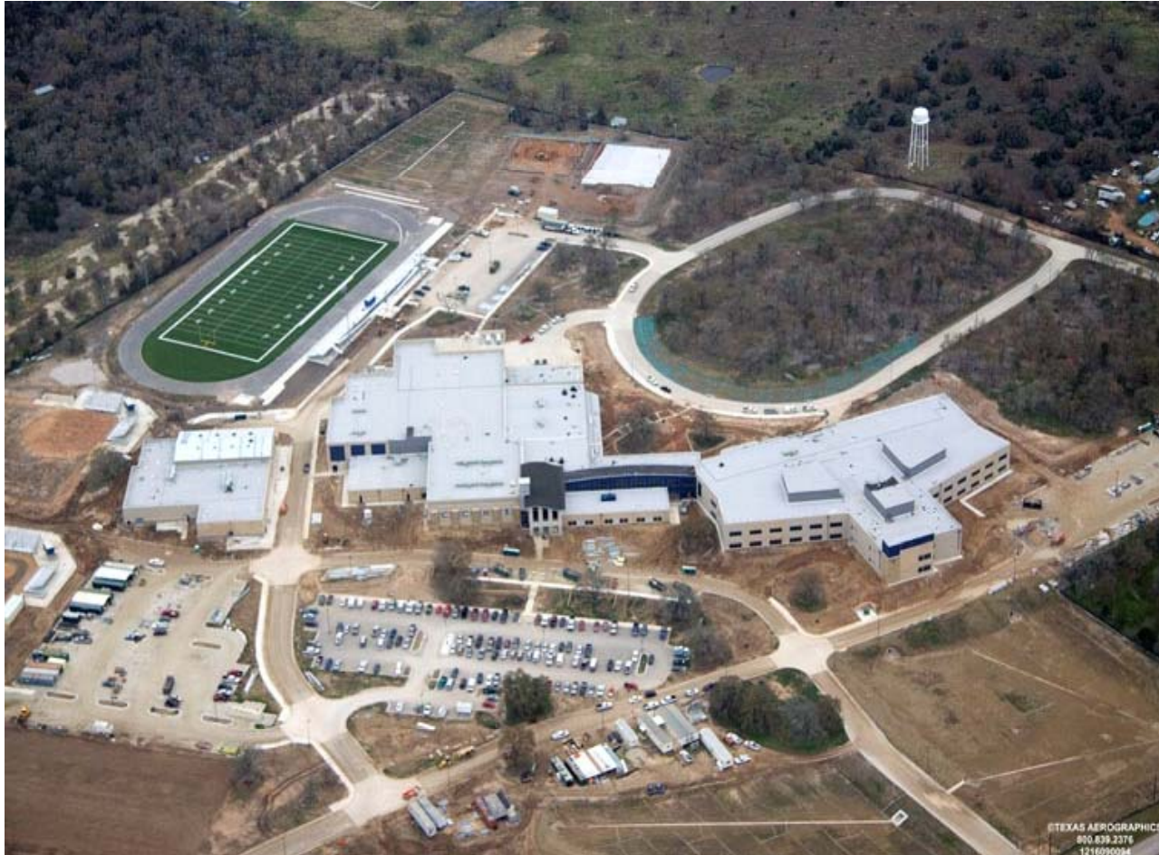
Aerial View of Site
