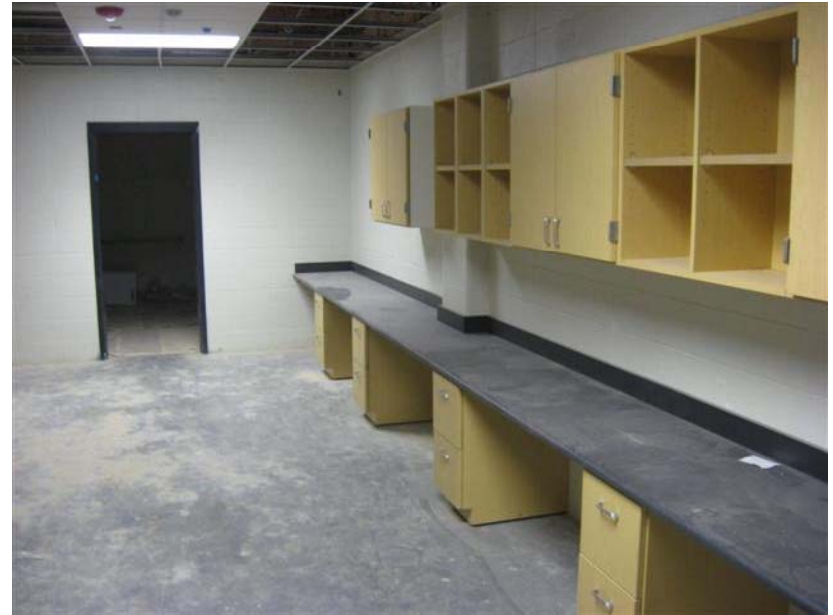
Millwork at Coach's Office
